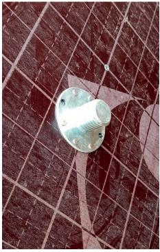
Whilst pouring concrete, the **positioning disc** is attached to the formwork on one side and to the climbing cone M24 on the other, helping to align it with the anchor plate embedded in the concrete.
