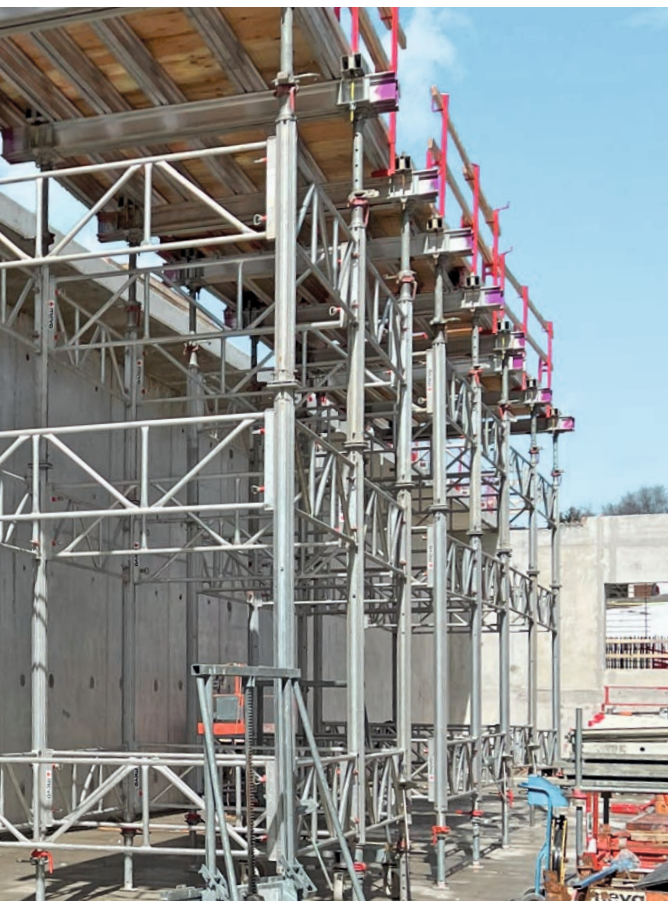
Left: 12'-0 x 8'-0 Imperial panels reduced the number of joints. Middle and right: Tables using the MEP aluminum shoring system were simply moved from pour to pour.
