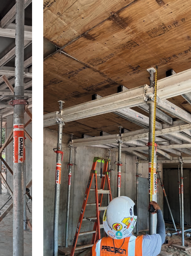
Formwork Superintendent Abraham Ramirez is pleased with the 7.5" Drop the HN drophead system has to offer.
