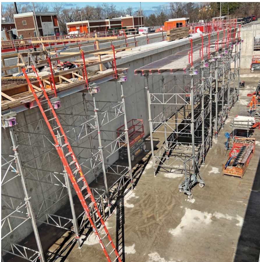
Left: 12'-0 x 8'-0 Imperial panels reduced the number of joints. Middle and right: Tables using the MEP aluminum shoring system were simply moved from pour to pour.
