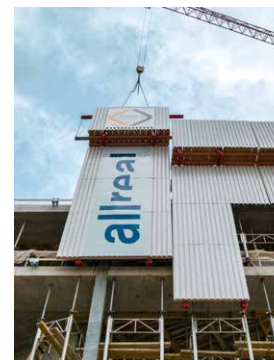
There are two options for advancing the screens to the next level: lifting by crane or by hydraulics
