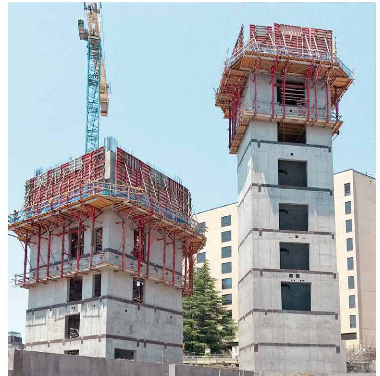
The KLK 230 climbing platform consists of climbing brackets, wall struts, planking, and handrails.
