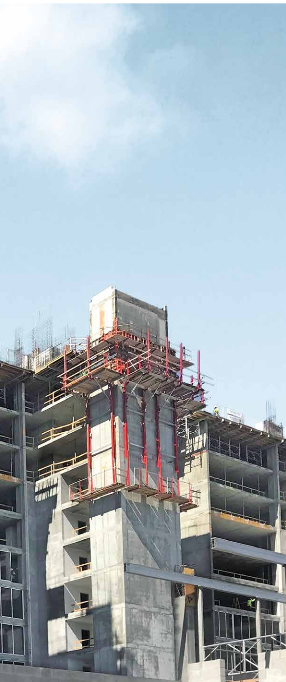
Even complex geometries with different sizes and offset structural elements can be easily achieved using the MGC-F guided climbing system.
