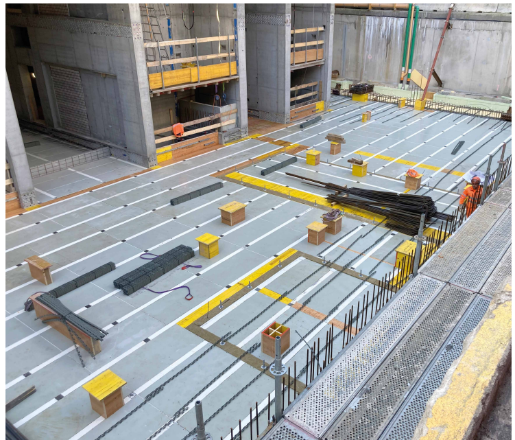
Left: The available space was very limited in the vicinity of the overhanging bracing slab. Right: All slabs were poured using MevaDec formwork.
