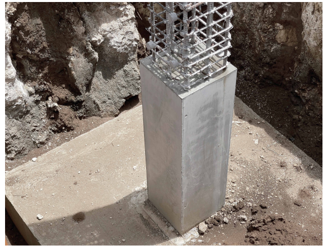
Above: The five-storey Boracay Convention Centre was completed by MEVBUILT as planned. Right: The building columns were erected using the lightweight, crane-independent AluFix wall formwork, impressing the construction team with their smooth, clean concrete surfaces.
