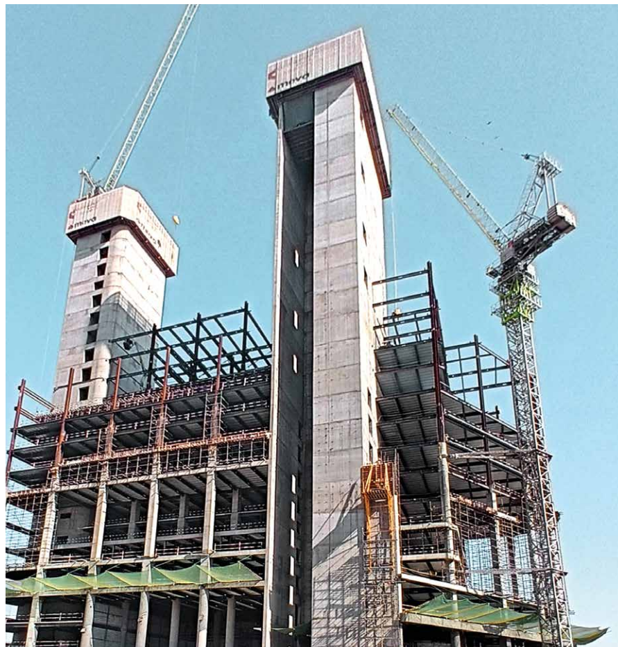
The MAC system saved time during the construction of the cores.
