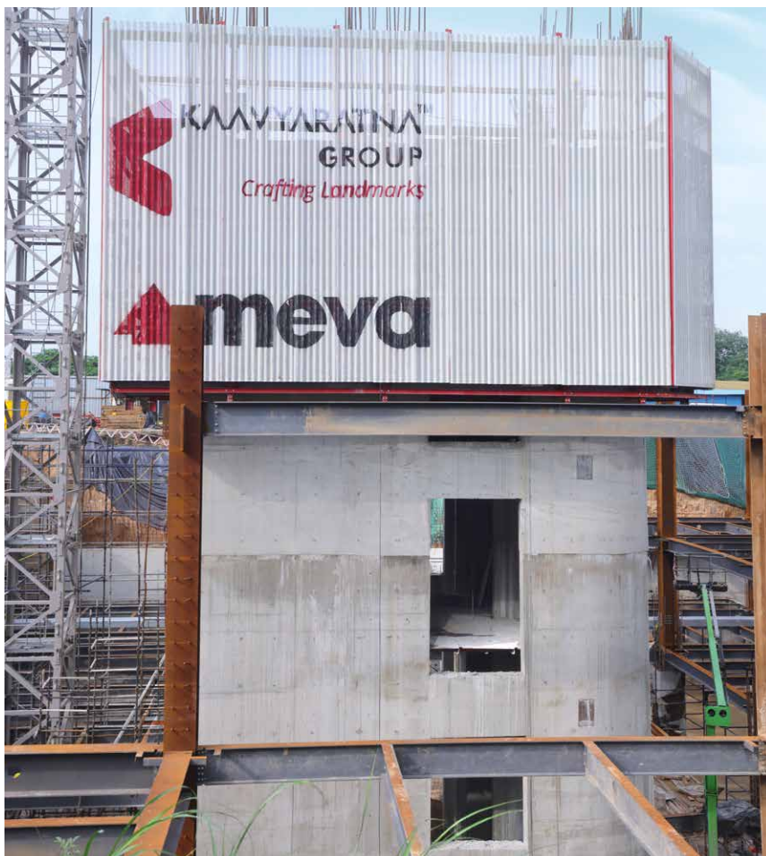
Left: The flexibility of MAC and MBS paid off in this project. Round corners on the cores were easy to form with this combination. Below: The external and internal walls of the cores were constructed using MBS wall and column formwork.
