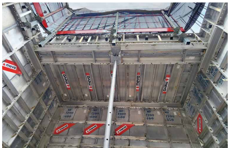
The slab formwork could be stripped early and prepared for the next use. MonoFix was used to pour the walls, slabs and stairs of the Alexa building.
