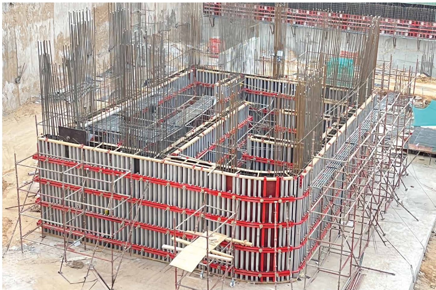
Left: The flexibility of MAC and MBS paid off in this project. Round corners on the cores were easy to form with this combination. Below: The external and internal walls of the cores were constructed using MBS wall and column formwork.
