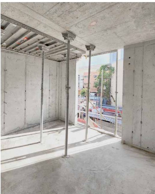
The slab formwork could be stripped early and prepared for the next use. MonoFix was used to pour the walls, slabs and stairs of the Alexa building.
