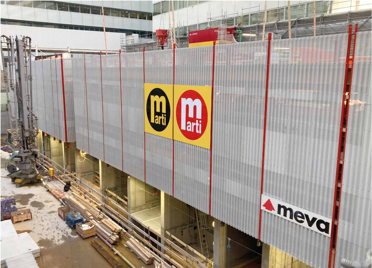
Top: The two high-rise cores climb concurrently out of the 22 m deep construction pit. The façades of the adjacent high-rise buildings are visible in the background. Left to right below: The bird's-eye view shows a tidy construction site typical of Marti in a restricted area. The support frames were used under the bracing slab and between the steel props. They were simply moved to their point of use on castors with a pallet truck.
