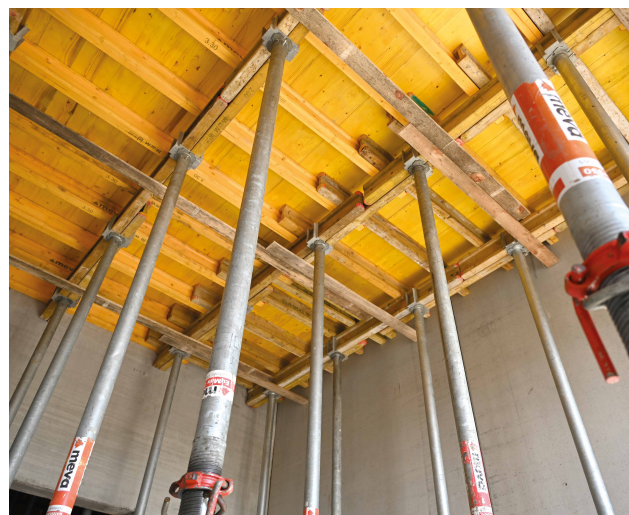
Clockwise from top left: EuMax props support freshly poured walls and the MevaFlex slab formwork. Prop heads and double girders were used under the formwork. The personnel profited from substantial freedom of movement under the slab formwork.
