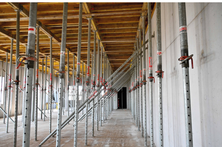
Clockwise from top left: EuMax props support freshly poured walls and the MevaFlex slab formwork. Prop heads and double girders were used under the formwork. The personnel profited from substantial freedom of movement under the slab formwork.
