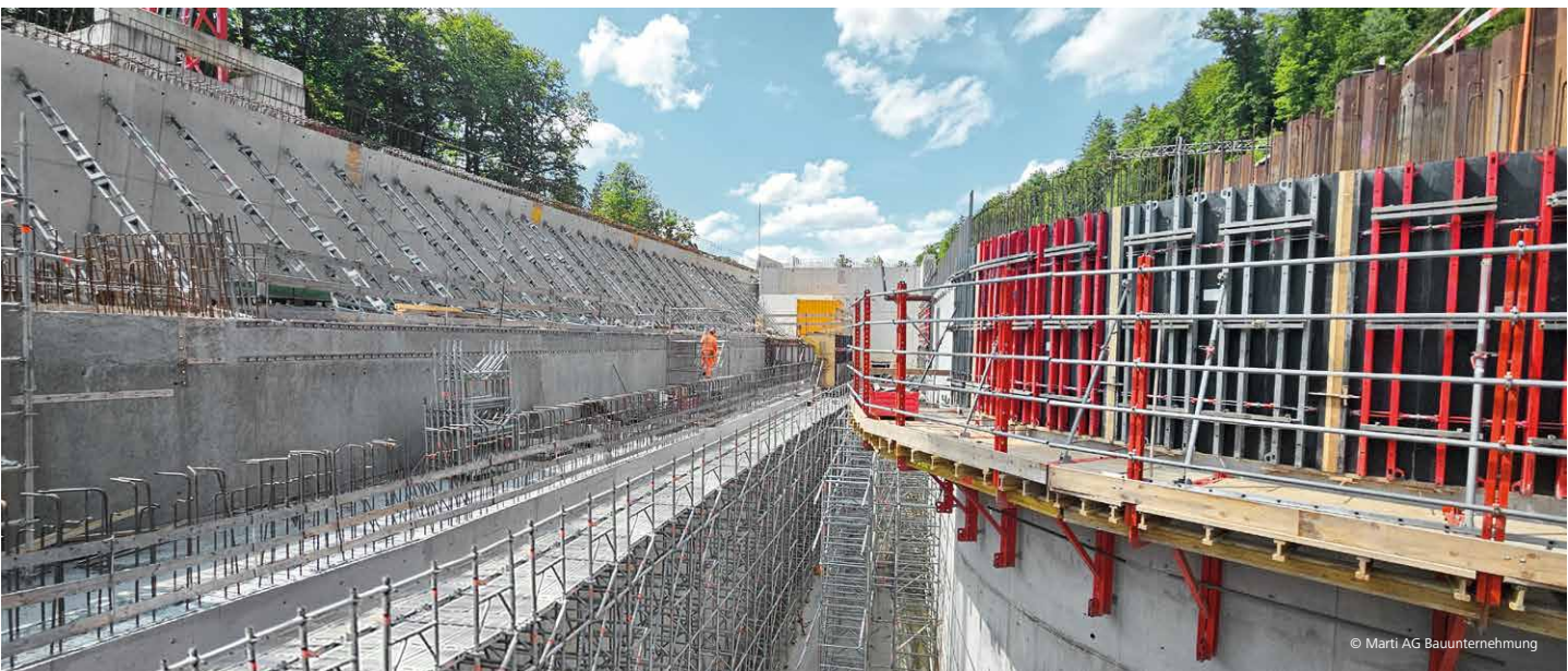
The sloping baffle wall can be seen top left and below this the longitudinal weir that enables the flood water to run over into the channel (in the middle). Between the round walls, the water is channelled into the underground pipes with a diameter of 6.6 m. The entire area is presently being roofed over and a plant building is being built on top of the tunnel's inlet structure. The final step will be to landscape the slab so that the inlet structure is almost completely invisible.
