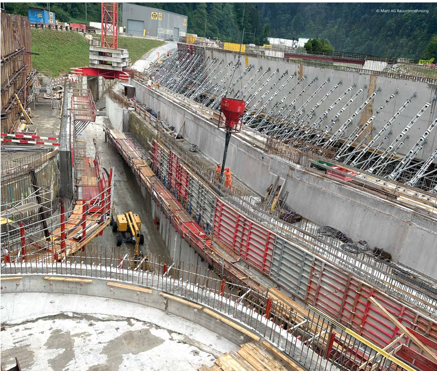
The sloping baffle wall can be seen top left and below this the longitudinal weir that enables the flood water to run over into the channel (in the middle). Between the round walls, the water is channelled into the underground pipes with a diameter of 6.6 m. The entire area is presently being roofed over and a plant building is being built on top of the tunnel's inlet structure. The final step will be to landscape the slab so that the inlet structure is almost completely invisible.
