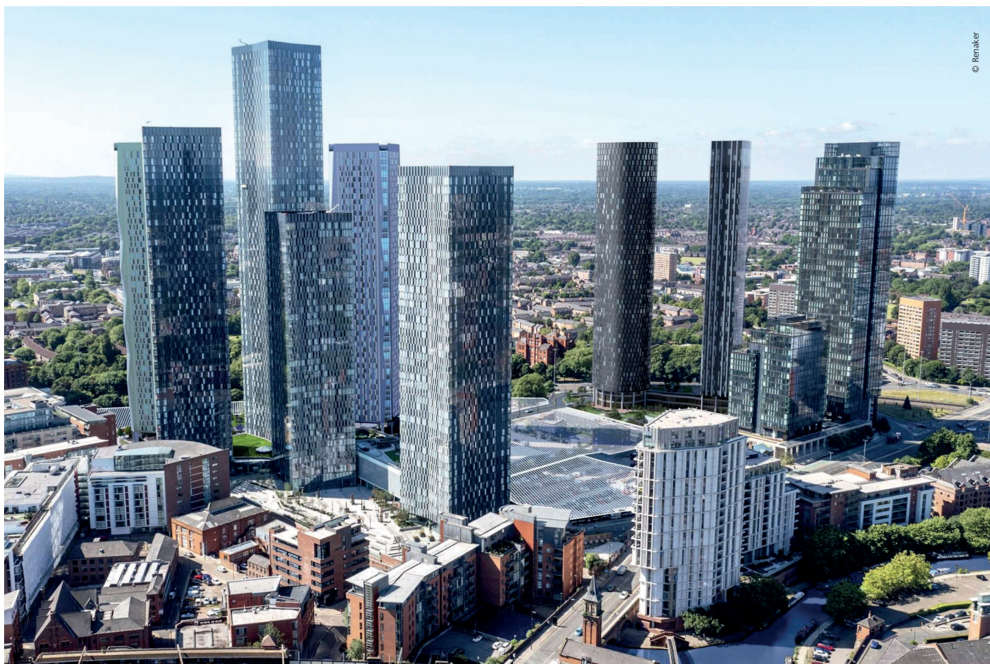
New Renaker construction project in the Jackson Street.
