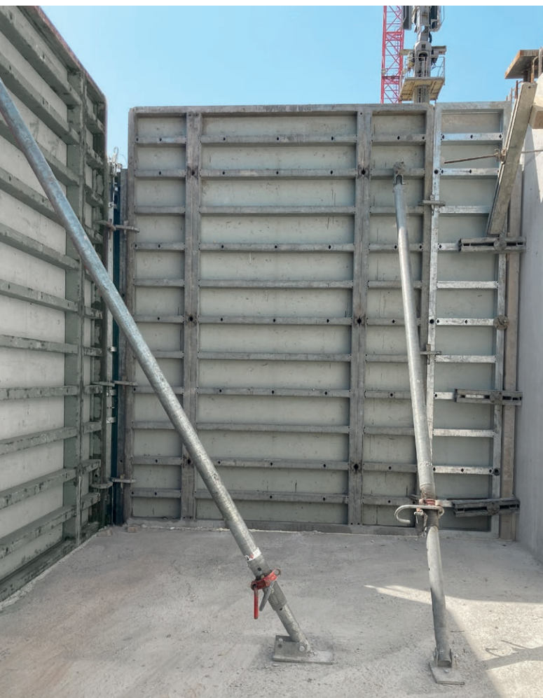
On the left: The high-performance Mammut 350 wall formwork allows for short pouring cycles. Top right: 23 bespoke shaft platforms were used for safe and comfortable work on the ten stairwell and elevator cores. Below: The shaft platforms were planned by MEVA and delivered to the construction site as pre-assembled units.
