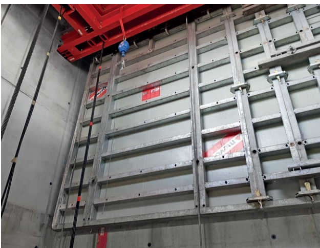
The hanging Mammut panels leave enough space for the rebars.
