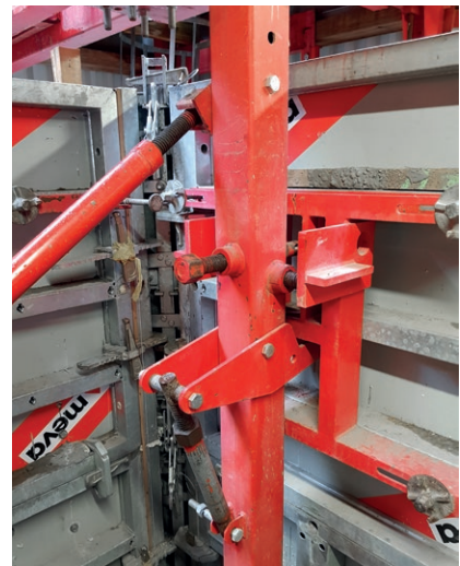
The formwork is precisely aligned by means of three-way adjustment.
