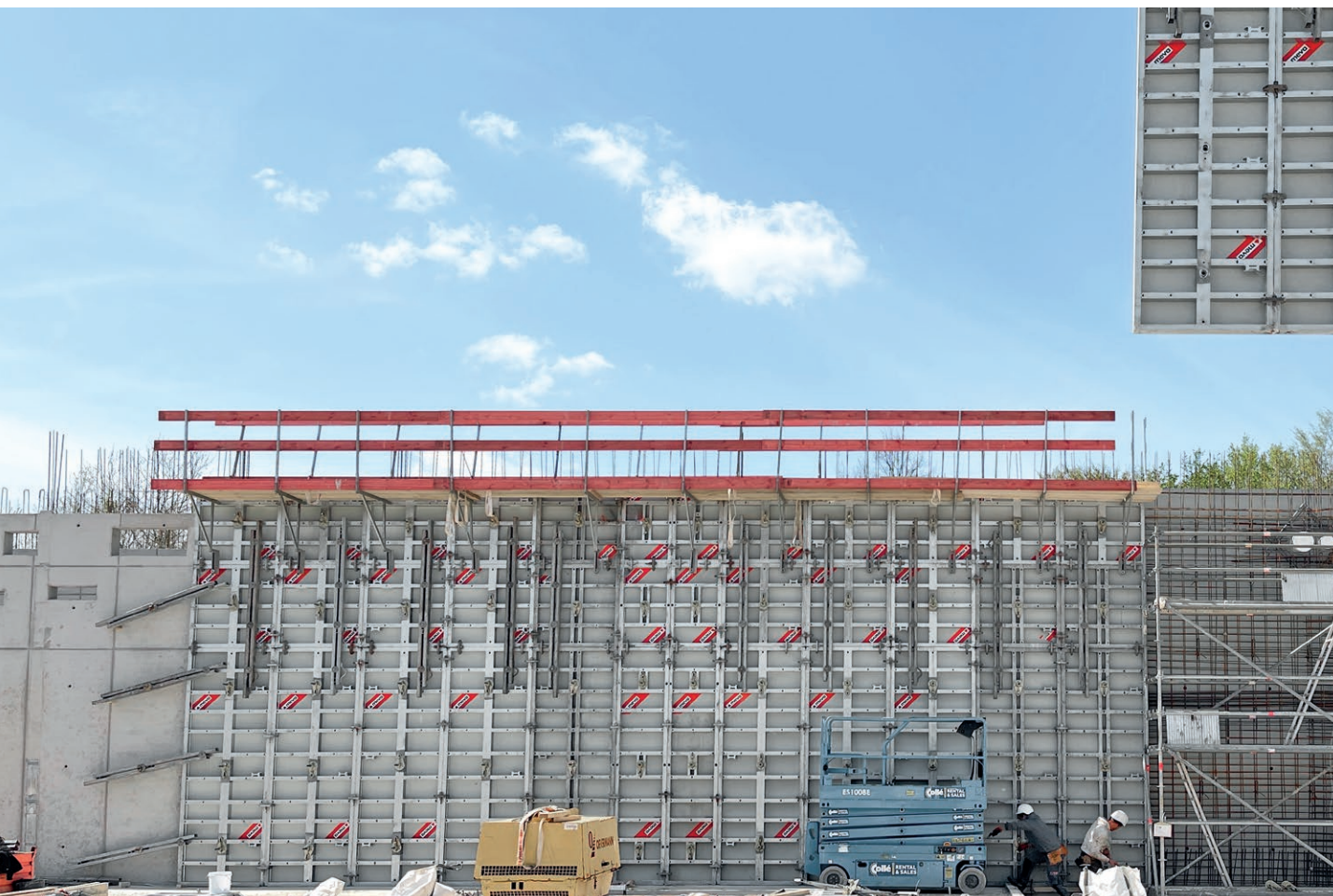
The height-extended formwork panels were transported by crane.
