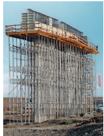
Clockwise from the top left: Several MEVA systems were combined. Circo circular column formwork was used to form the outer corners. Special wooden formwork panels suitable for multiple use were employed, here for the pier heads. The MEP shoring tower was adapted without problem to suit the elliptically shaped piers; the result: absolute perfection!
