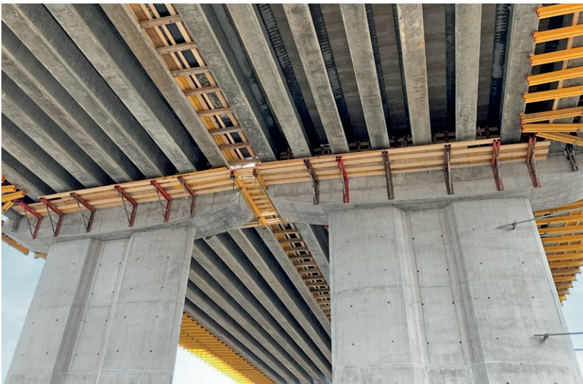
Clockwise from the top left: Several MEVA systems were combined. Circo circular column formwork was used to form the outer corners. Special wooden formwork panels suitable for multiple use were employed, here for the pier heads. The MEP shoring tower was adapted without problem to suit the elliptically shaped piers; the result: absolute perfection!
