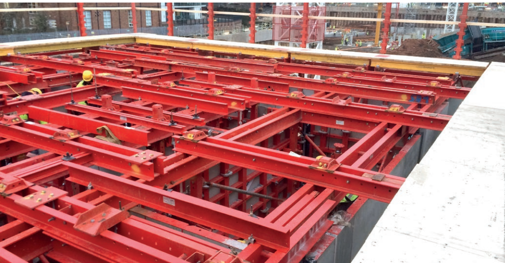
The formwork is suspended from the steel grid.
