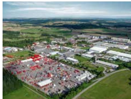
MEVA's headquarters is located in Haiterbach in the Northern Black Forest. The company also operates 40 sites on five continents.
