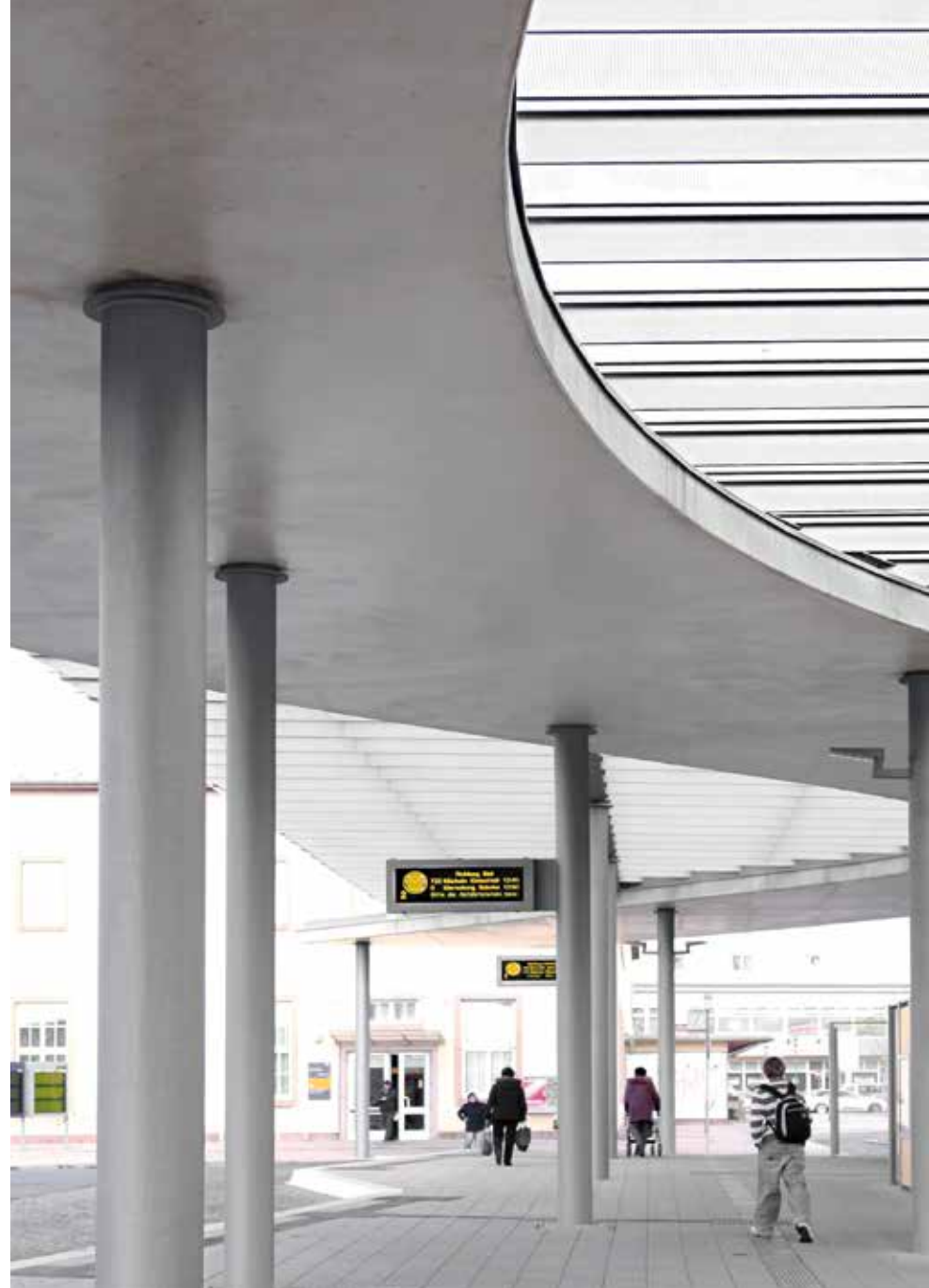
Bus station in Merseburg, Germany: Optimally shaped, precision-cut and welded alkus facings were used to cast a jointless, 760 m 2 , SB4-grade fair-faced concrete slab.
