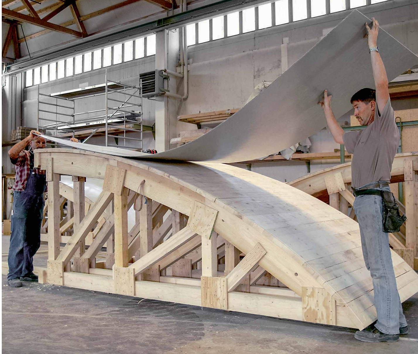
Large-format 6 mm (GM) alkus all-plastic facing on a wooden substructure.
