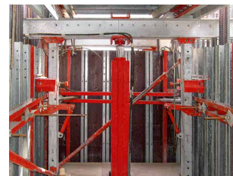
High-performance hydraulic system of the MAC automatic climbing system allows a stroke of 4.5 metres (20 t per cylinder).
