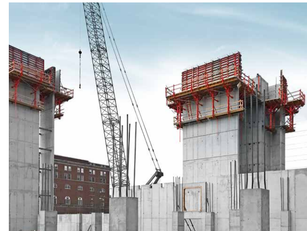
The KLK 230 climbing system consists of climbing brackets, wall struts, planking and handrails.
