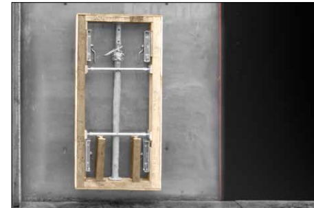
Box outs Magnets used to attach box outs and triangular fillets.
