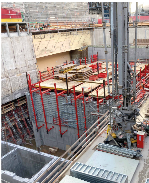
Above left: The MAC unit is already being assembled for the northern core on the lowest, completely concreted storey. After reaching ground level, the work makes rapid progress upwards with the construction of the uniform upper floors.
