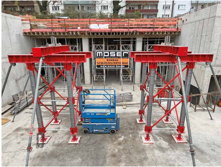
Above: The two MEKit support towers were quickly set up on the construction site in Karlsruhe. Below: The basement with the steel truss beam after completion. Photo on next page: An MEP shoring tower can be seen in the background on the right.
