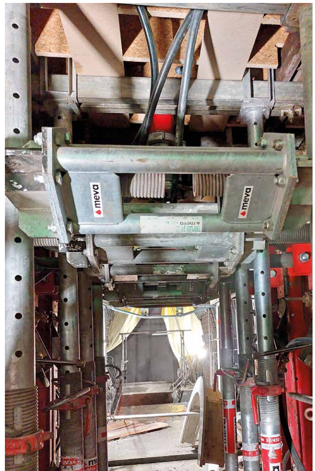
Top: Special formwork at the intersection between the supply cross-passage and the vertical shaft. Bottom right: The folded-in vault formwork entering the emergency cross-passage – high-precision work! Bottom left: The formwork for the intermediate and connection blocks is ready for use and the transport carriage with hydraulics has been moved back. Bottom right: The formwork for the supply cross-passage required innovative ideas.
