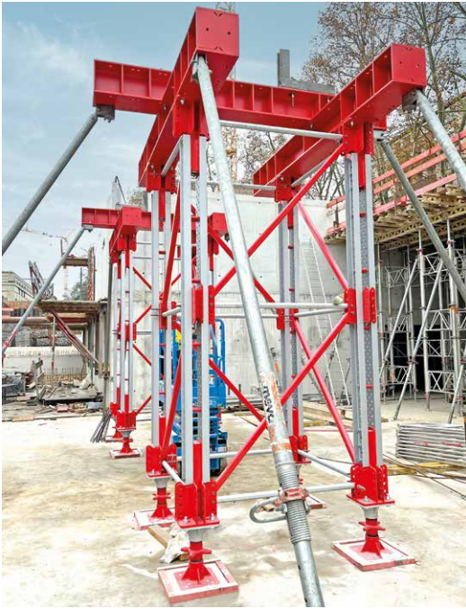
Above: The two MEKit support towers were quickly set up on the construction site in Karlsruhe. Below: The basement with the steel truss beam after completion. Photo on next page: An MEP shoring tower can be seen in the background on the right.
