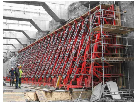
Supporting single-sided formwork up to a height of 13.50 m.
