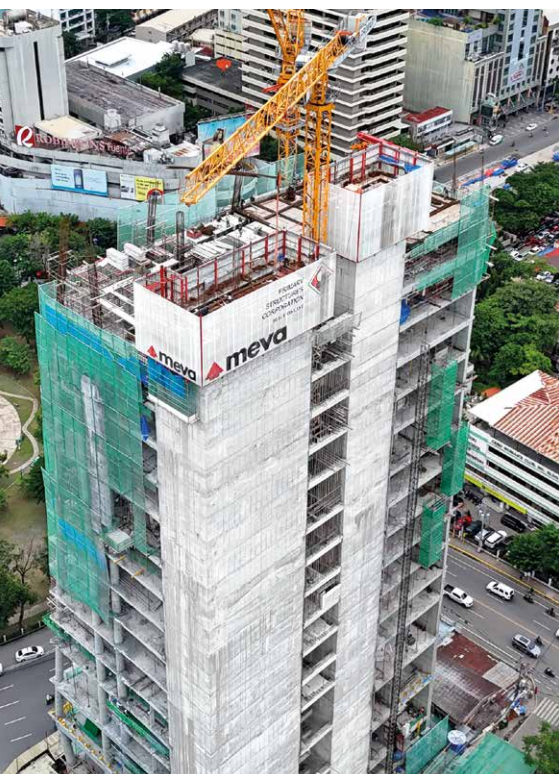
The central location in Cebu City made logistics difficult. Right: The cooperation between Primary Structures Corporation and MEVA went smoothly. Below: The enclosed MAC climbing systems protected the workers from wind and weather.
