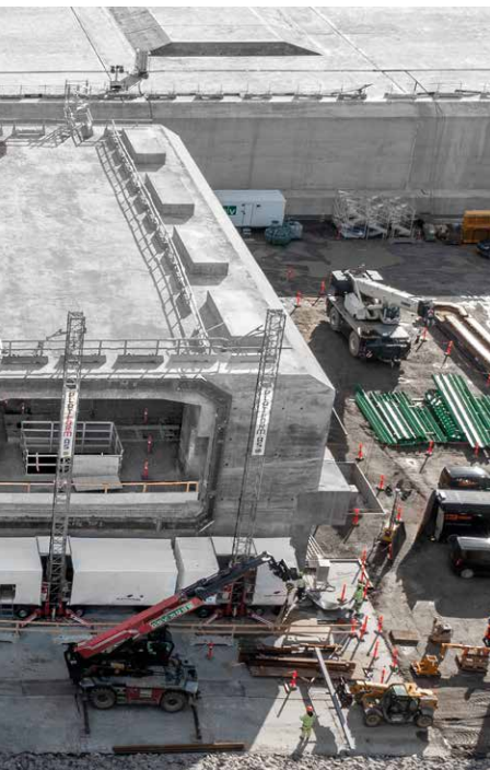
Above, from the left: The work harbour with six production lines and three dry docks. – A special tunnel element (SPE) is driven out to the dry dock. – The floating gate with eight chambers in one of the three dry dock portals with 21 m high abutments.
