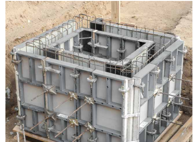
By using inside and outside corners as well as continuously adjustable hinged corners, it is possible to form all angles between 0° and 180°.
