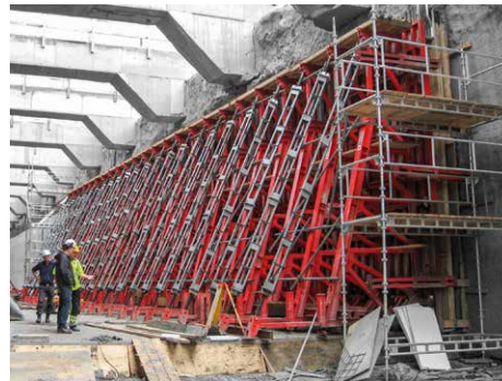
Supporting single-sided formwork up to a height of 13.50 m.
