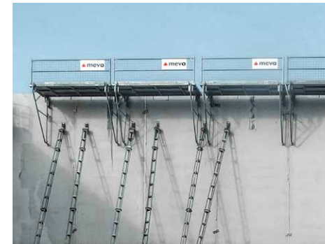
With precast wall constructions, the LAB 130 system is used in conjunction with the formwork connector head to create a safe working and pouring platform.
