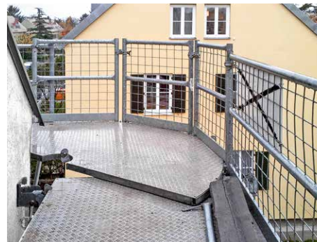
Crescent-shaped corner platforms simplify planning.
