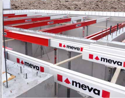
Slab formwork systems
