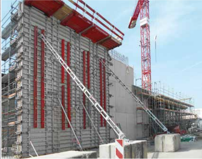
Wall formwork systems
