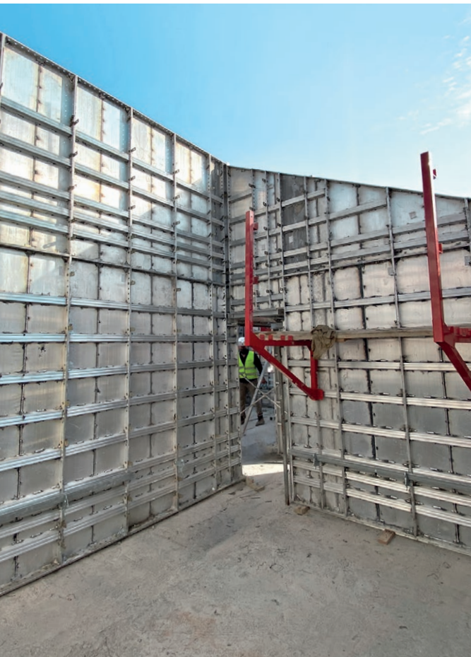
The formwork proved its worth right from the start.
