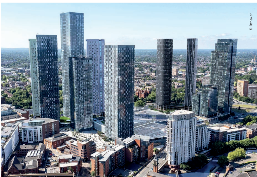
New Renaker construction project in Jackson Street.
