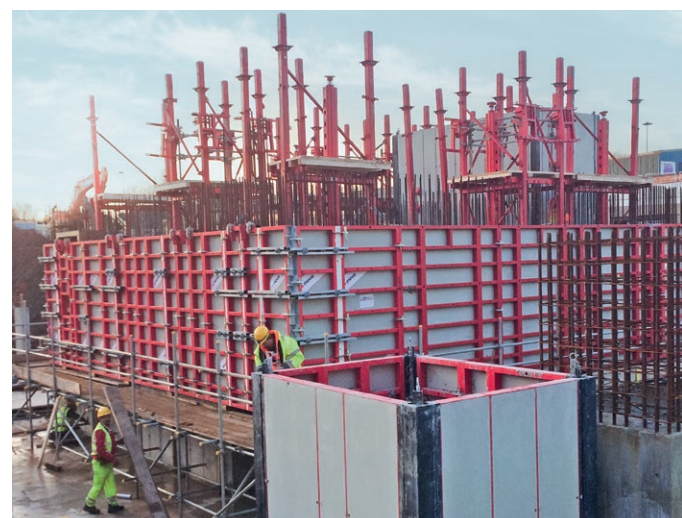
Inside-formwork boxes were assembled next to the core and then lifted into place.
