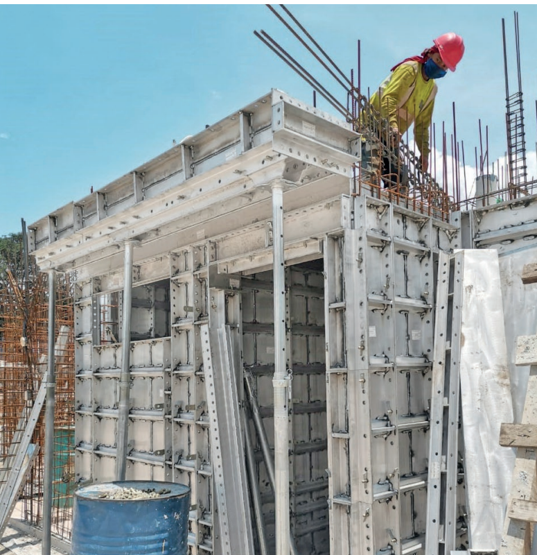
Windows and doors are simply cut out while balconies, columns and beams can be formed as required – all with just one formwork system.
