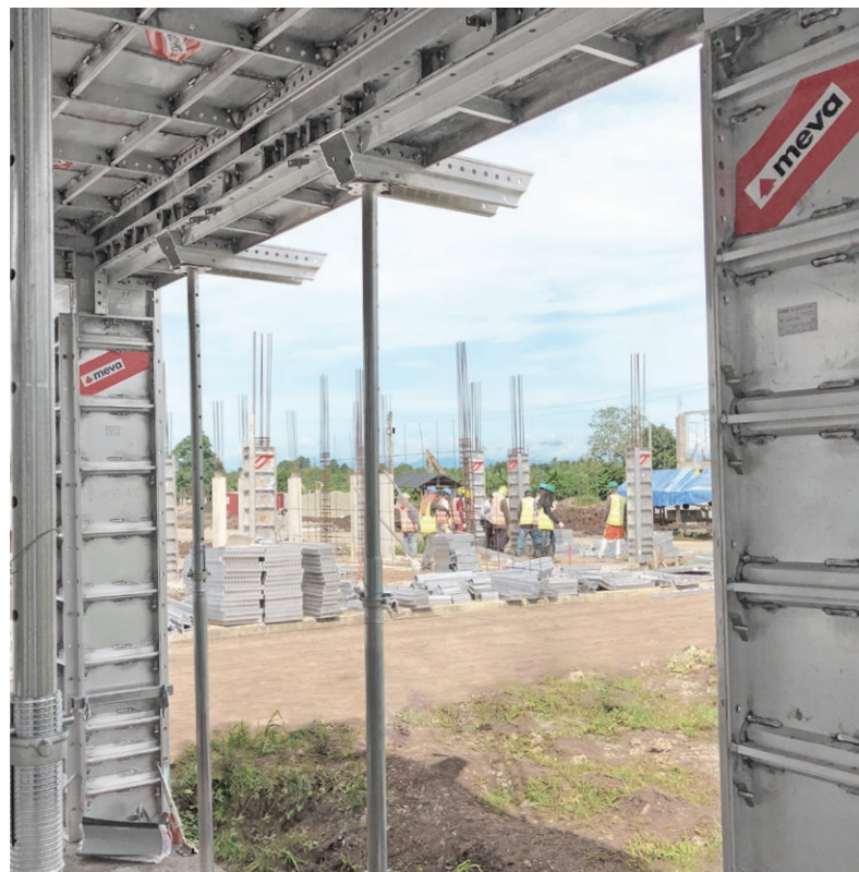
Windows and doors are simply cut out while balconies, columns and beams can be formed as required – all with just one formwork system.
