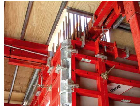
The wall formwork panels are suspended, can be moved back manually, and allow the formwork to be opened quickly and easily.
