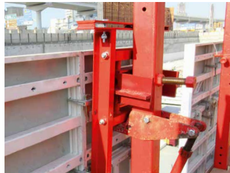
The 3-way adjustment allows for utmost precision. The suspended formwork can be moved and adjusted manually in three directions and can thus be quickly and easily adapted to suit the geometry of the building.
