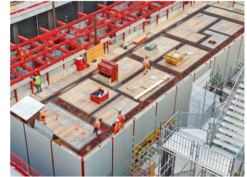
The top deck of the MAC is free of jacking masts, thus ensuring an optimum level of safety, a minimum risk of accidents and more storage space.
